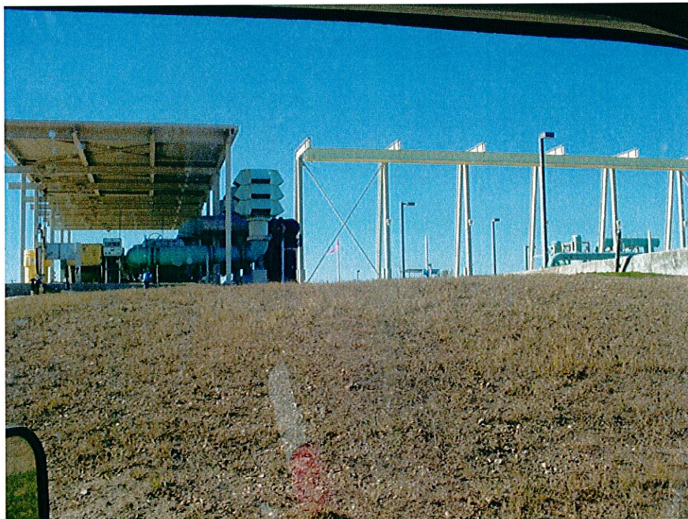
Site Photo 8 – Vicinity of Test Boring B-7
