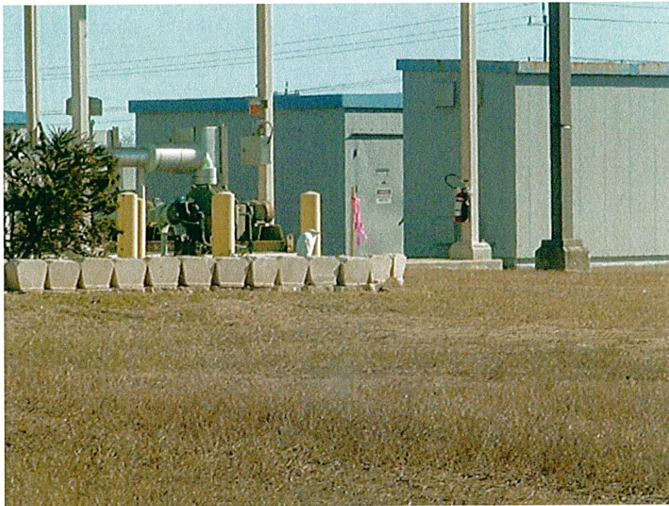
Site Photo 4 – Vicinity of Test Boring B-3
