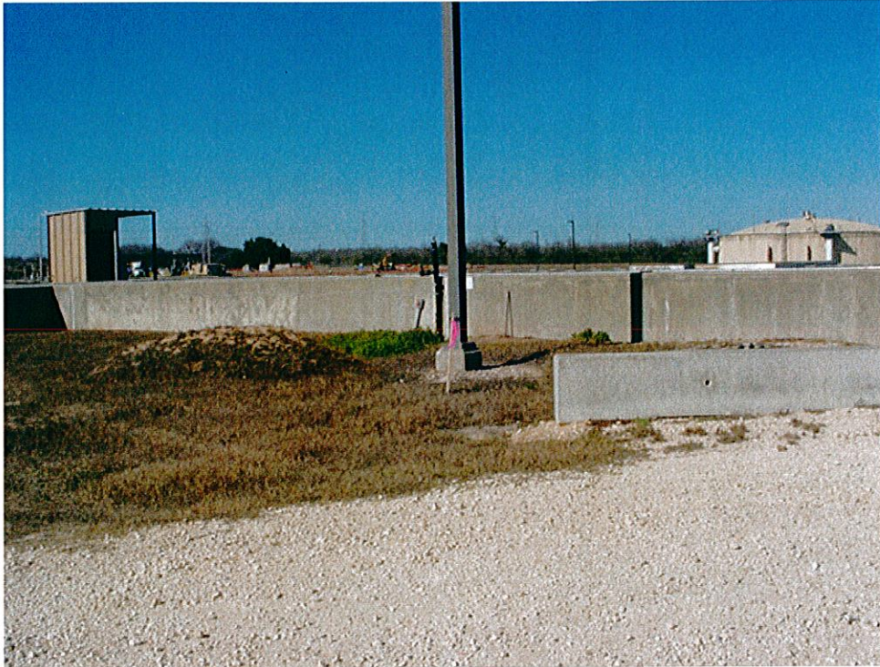
Site Photo 1 – Vicinity of Test Boring B-1
