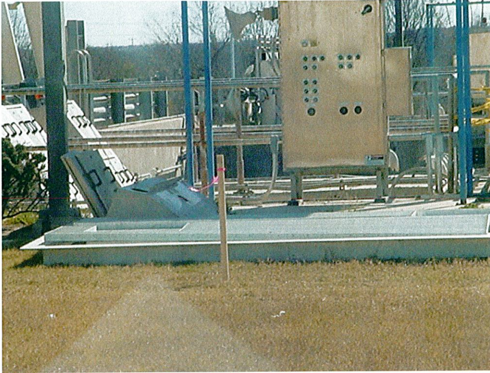
Site Photo 3 – Vicinity of Test Boring B-2
